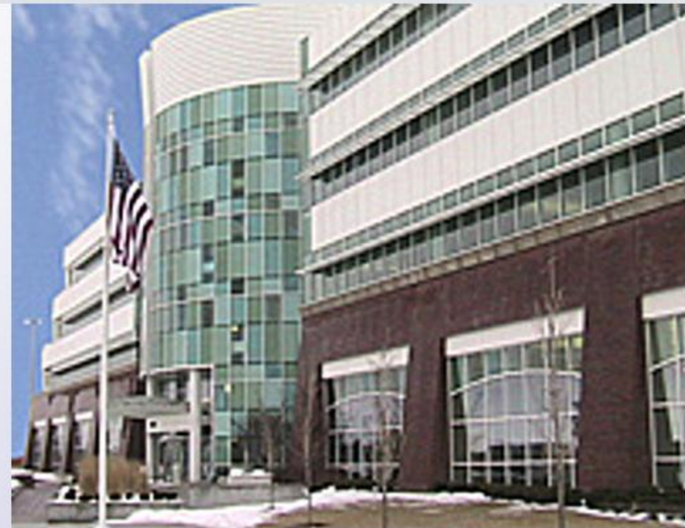
Acheson Ventures Office Building, Port Huron, MI Contractor: American Glass & Metals Corp.
